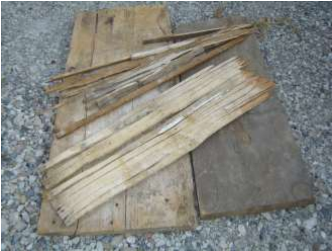
Split and spread like an accordion, this Scarborough farmer-made wood lath was used for plastering walls in the mid 19th century.
